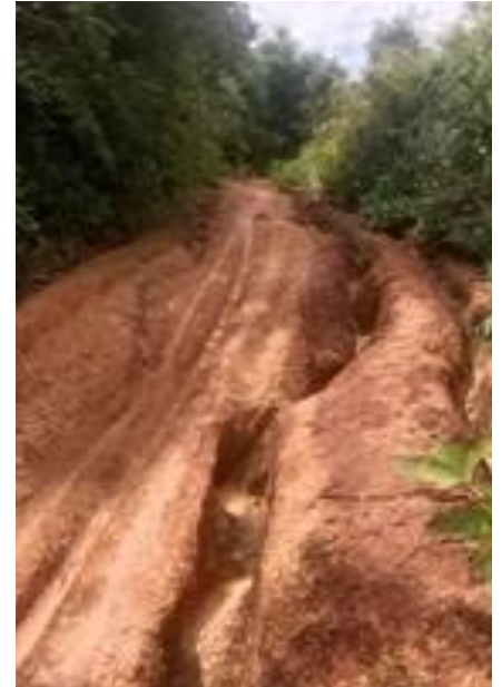
Condition of the dirt road connecting Ong Jangking to the main road before repairs. Long stretches of road had been eroded during the rainy season.
