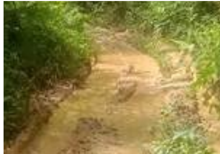
Condition of the dirt road connecting Ong Jangking to the main road before repairs. Long stretches of road had been eroded during the rainy season.
