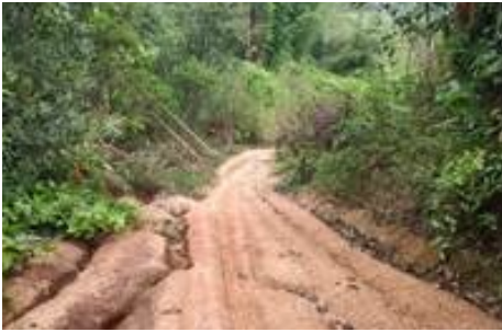
Condition of the dirt road connecting Ong Jangking to the main road before repairs. Long stretches of road had been eroded during the rainy season.
